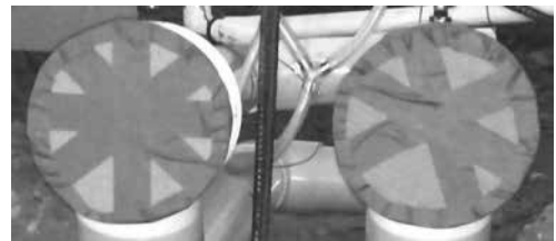
Figure 9 Taped Jet Housings
