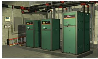
Hybrid system using 2-MVB's and 1-XTherm
