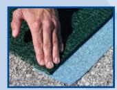
Place matting over the adhesive and apply pressure along length of reinforcement strip.
