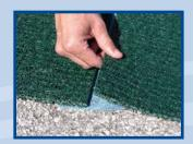
Begin to align loose mat into place along the exposed portion of reinforcement strip.
