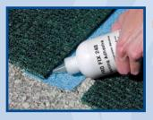
Apply another bead of Pro Fix 240 Seam Adhesive along the other half of reinforcement strip. Be sure adhesive is also applied along the edge of mat already in place.
