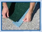
Once all matting is in place and lying flat, apply reinforcement strips directly beneath all areas to be seamed.
