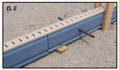
**D.** Install the top cap, making sure to "half-lap" the top past the joints to insure rigidity. Add additional stakes on either side of the drain to temporarily support the drain during the pour.
