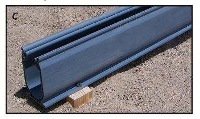
**C.** Using nails or sheet rock screws, fasten the drain to the 3 inch stakes that have been set to grade.
