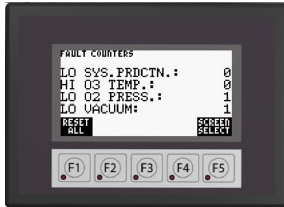
Fault Counters Screen
