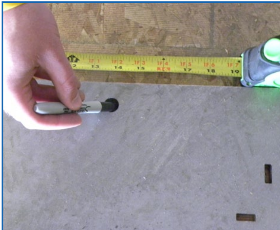
MARK THE FOUR MOUNTING HOLES
