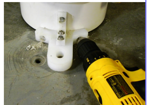
MATCH-DRILL OTHER HOLES (CENTER BOLT INSTALLED)
